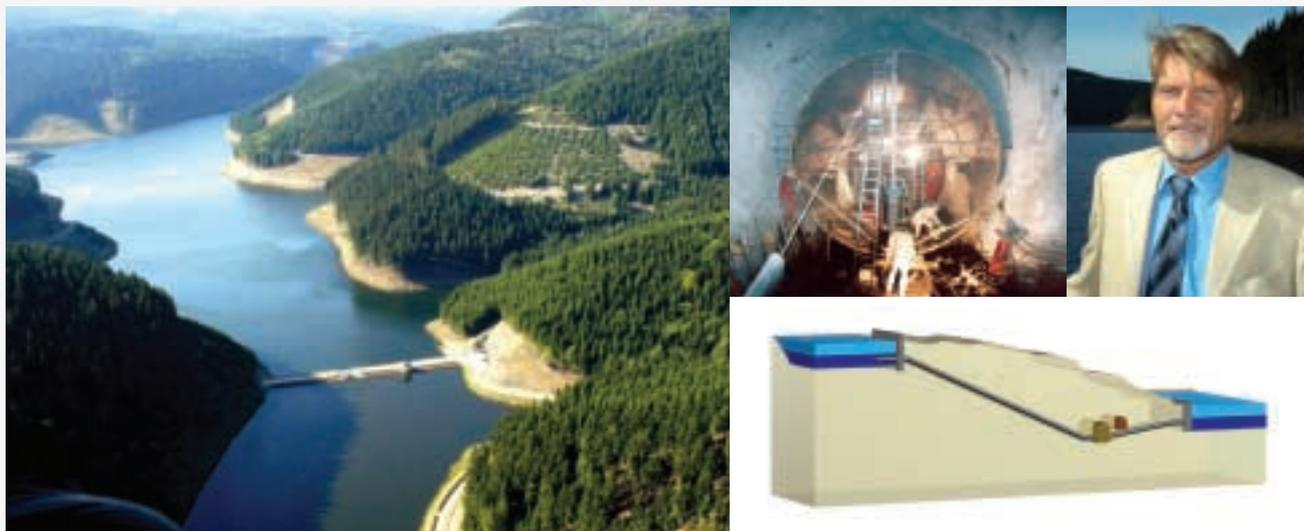
"In the Goldsthal power pumped storage plant, the water passes from one water storage dam to the other through a tunnel. Together, both water storage dams hold 30 million cubic metres," explains Project Manager, Wolfgang Bogenrieder.
