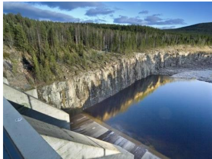
Power Generation – Generation
