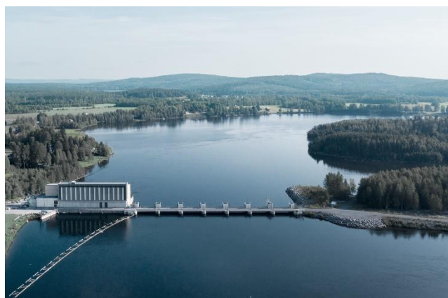
Vittjärv hydro power plant in Sweden
