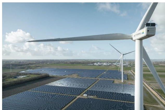
Haringvliet energy park, the Netherlands
