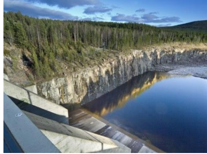
Power Generation – Generation
