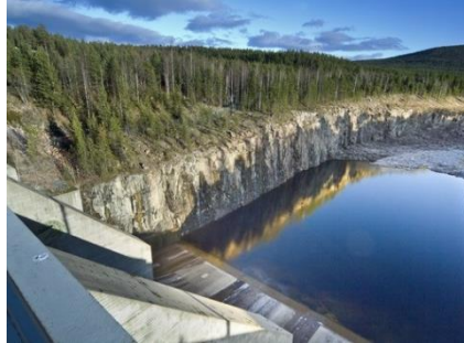
Power Generation – Generation
