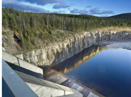
Power Generation – Generation
