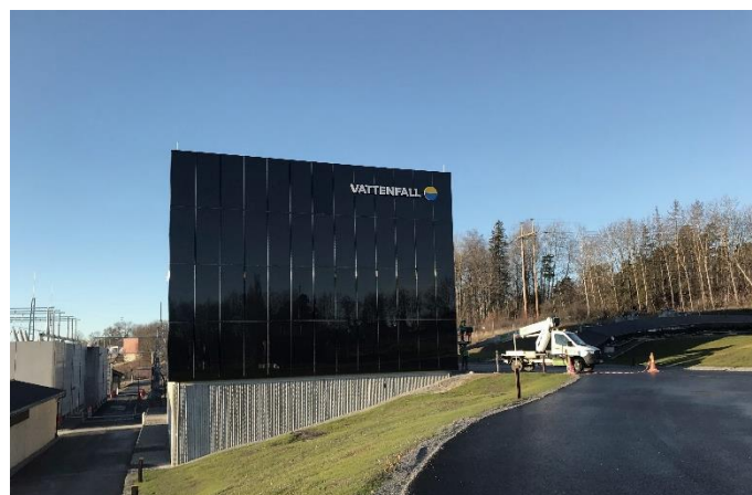
Vattenfall's transformer station in Järva, Stockholm Sweden
