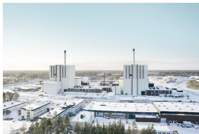
Forsmark nuclear power plant, Sweden
