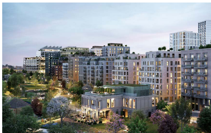
London Brent Cross South - Vattenfall's first district heating network in the UK.
