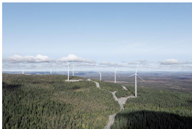
Blakliden Fäbodberget onshore wind farm, Sweden
