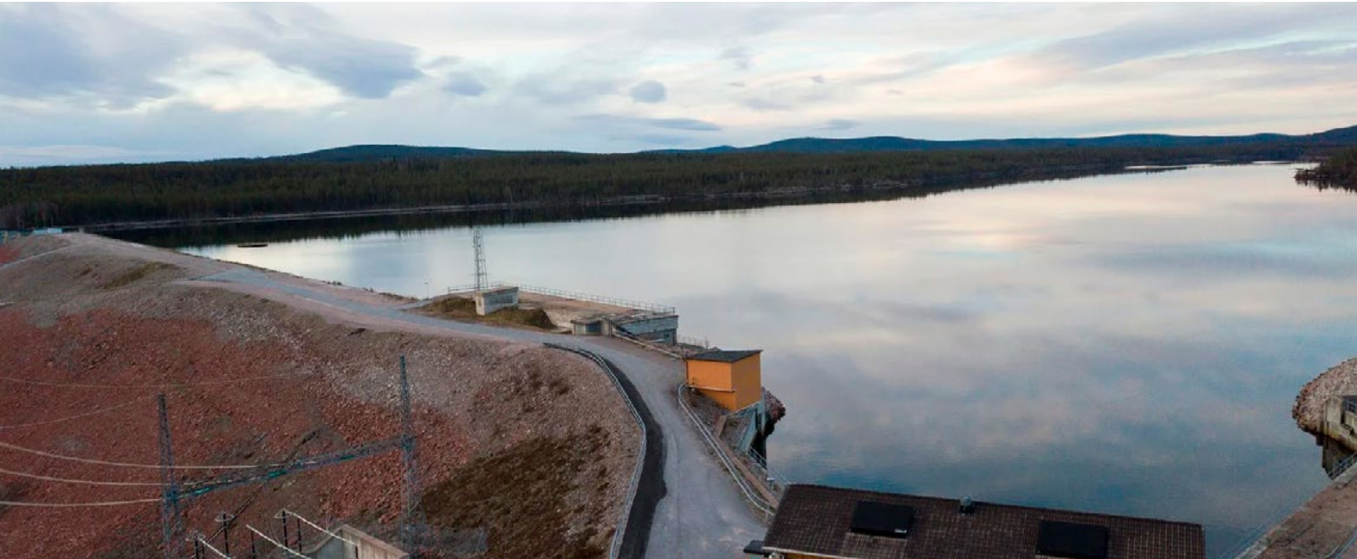
Harsprånget G3 630 MSEK Investment in new turbine for Harsprånget hydropower plant. Planned completion 2028.
