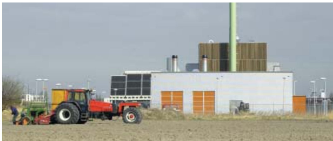
De biomassa-centrale in Lelystad.
