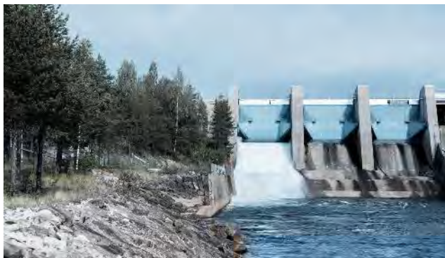
Laxede power plant, Sweden
