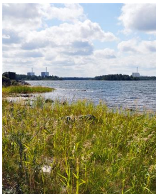
Forsmark nuclear power plant
