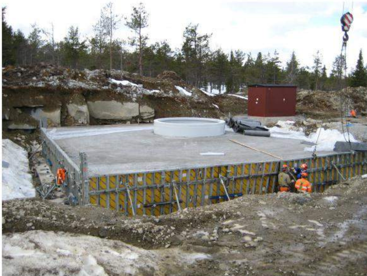
Figur 5:3. Gravitationsfundament
