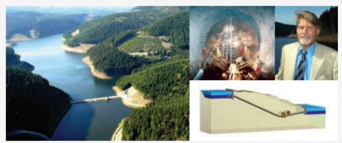
"In the Goldsthal power pumped storage plant, the water passes from one water storage dam to the other through a tunnel. Together, both water storage dams hold 30 million cubic metres," explains Project Manager, Wolfgang Bogenrieder.
