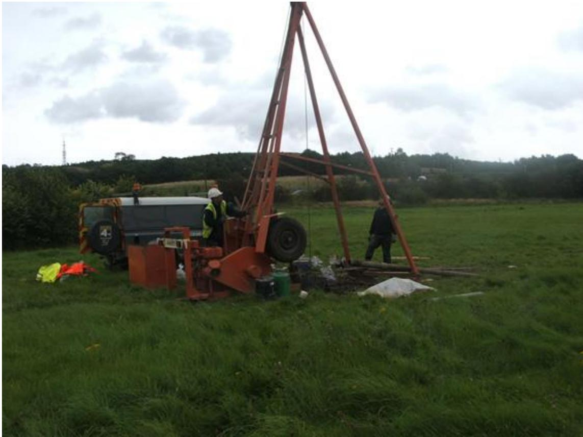
Fig 1. Picture of a borehole drill rig of the type that will be deployed locally.
