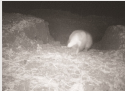
Construction management in action! Badger using a ramp excavated in a cable trench to ensure animals do not get trapped within the open trench.
