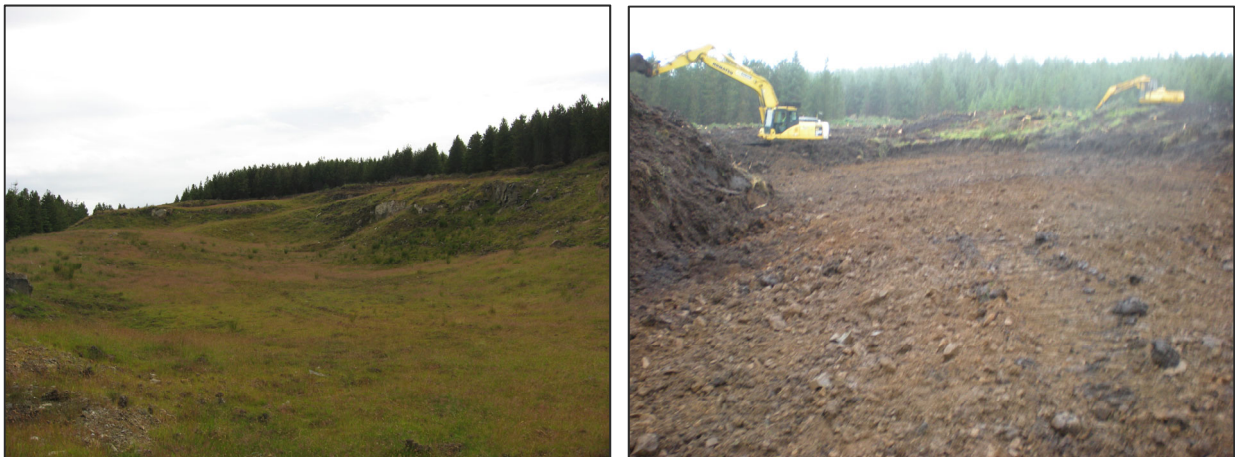
Plate 12.1 Typical Borrow Pit Reinstatement (18 months after completion of borrow pit operation)
