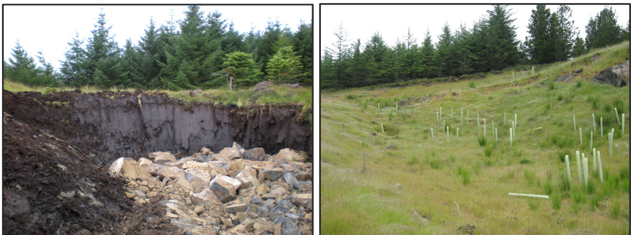
Plate 4.1 Photograph of typical borrow pit restoration, 18 months after completion of borrow pit operation
