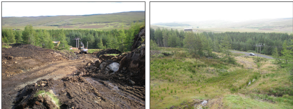
Plate 12.2 Typical Borrow Pit Access Road Reinstatement (18 months after completion of borrow pit)
