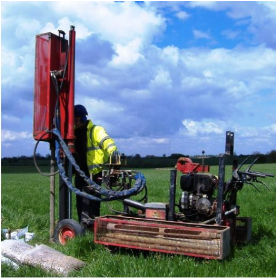
Fig 3. Window sample drilling rig
