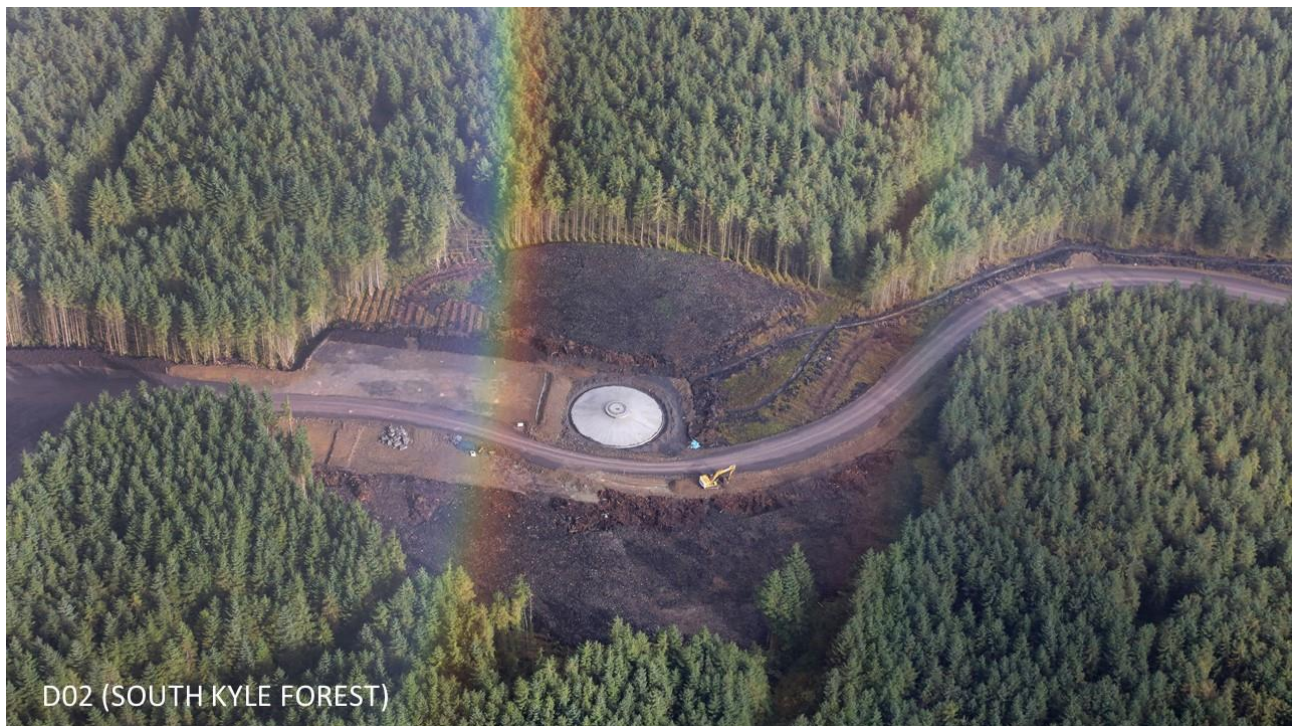
Diagram 3.1: Concrete turbine foundation (South Kyle Wind Farm)
