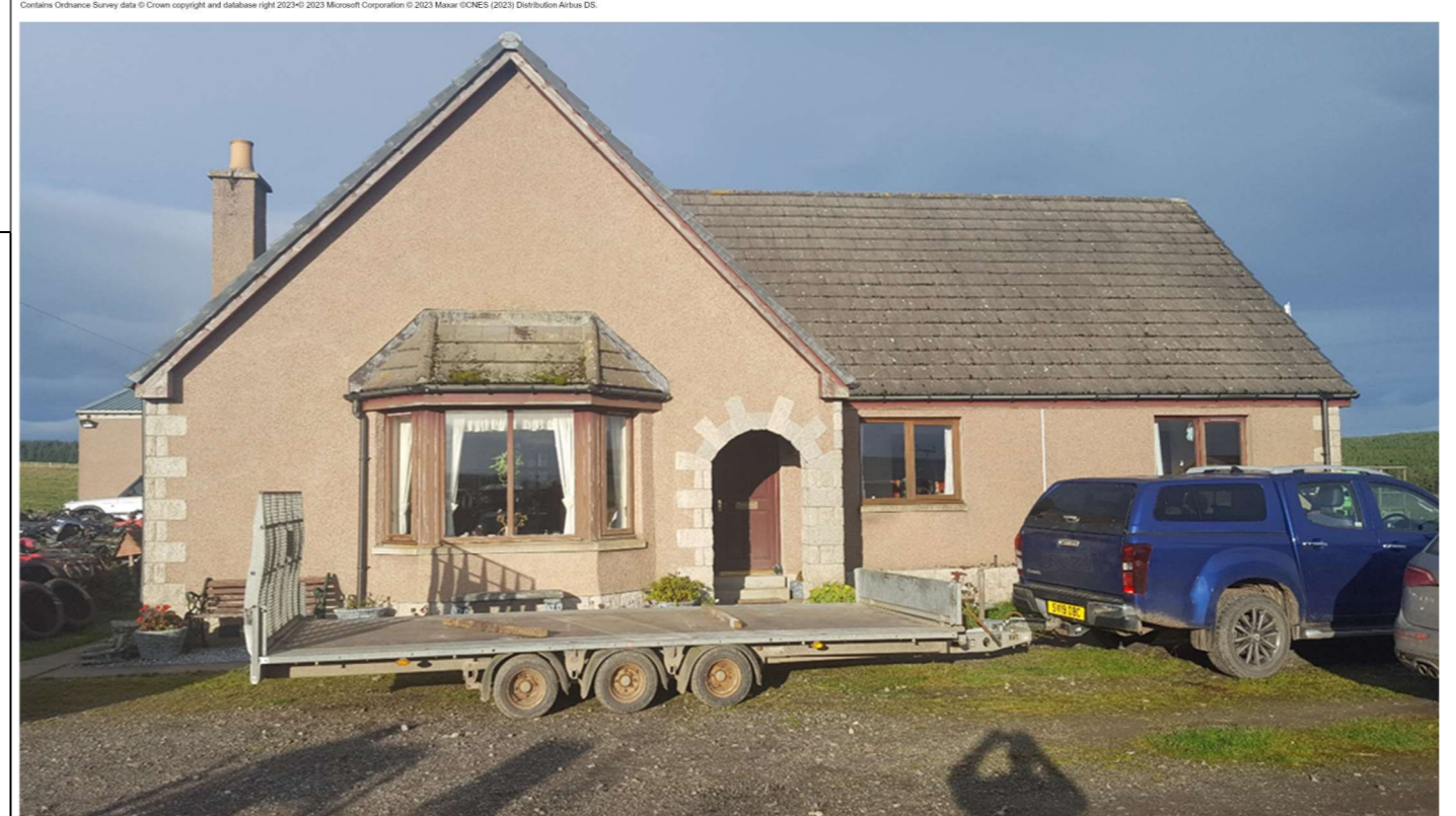
View of south facing façade and main outlook from the dwelling
