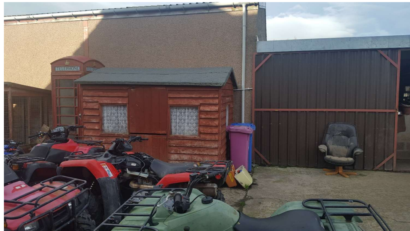
View from the north facing façade and side entrance to the dwelling showing large sheds that interrupt views
