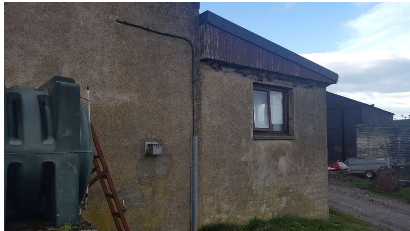
Small window on eastern façade of extension
