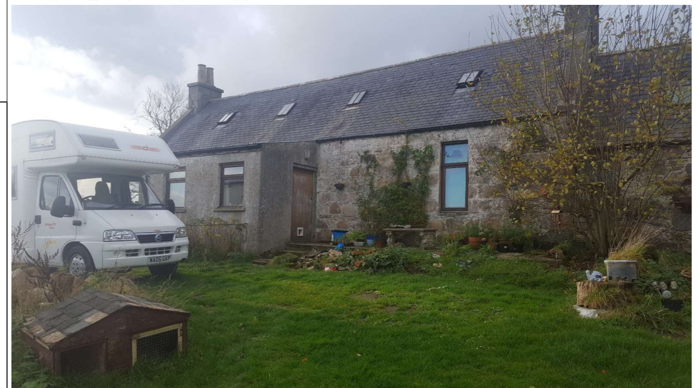
View of eastern façade
