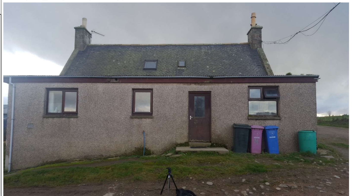
View of northern façade
