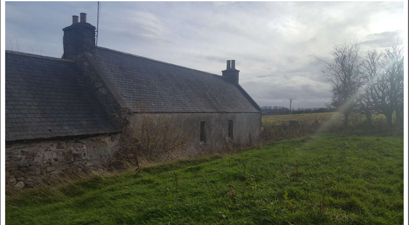
View of western façade
