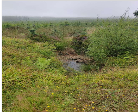
Photograph 3-1 Drain flowing out from under track, down side of plantation
